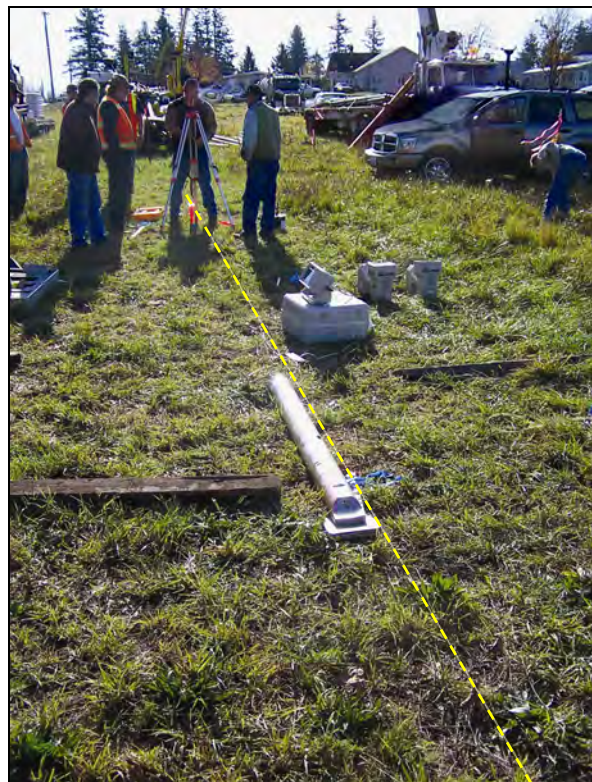
Aligning Drill to Marked Borepath
