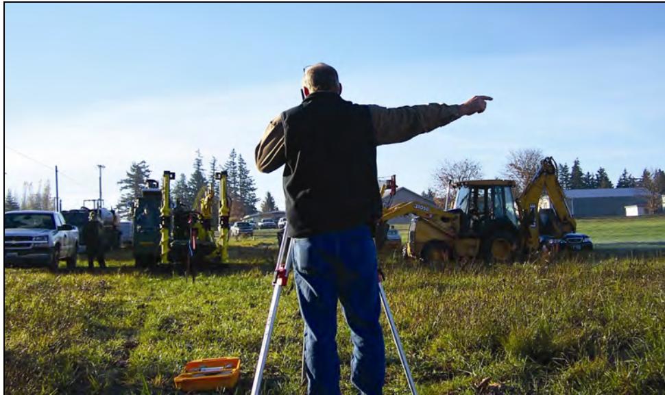
Aligning Drill to Marked Borepath
